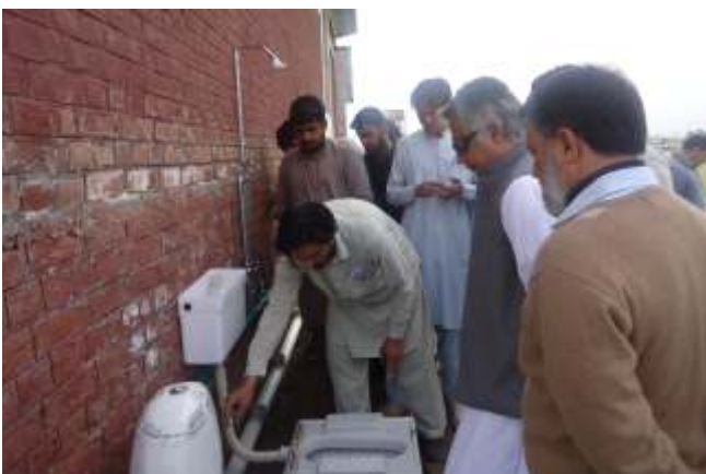
Plumbing course trainees briefing CE BEFARe about models made by trainees during training
