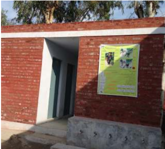
Newly constructed washroom facility at GGPS Kagaan
