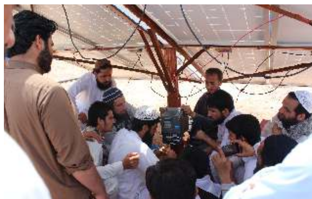
BEFARe trainees connecting cables during installation of solar panels for water pumps
