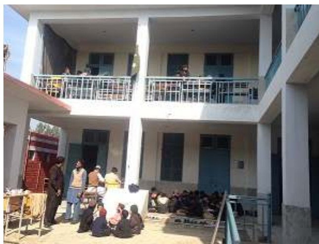
A view of newly constructed class rooms at GPS Kagaan
